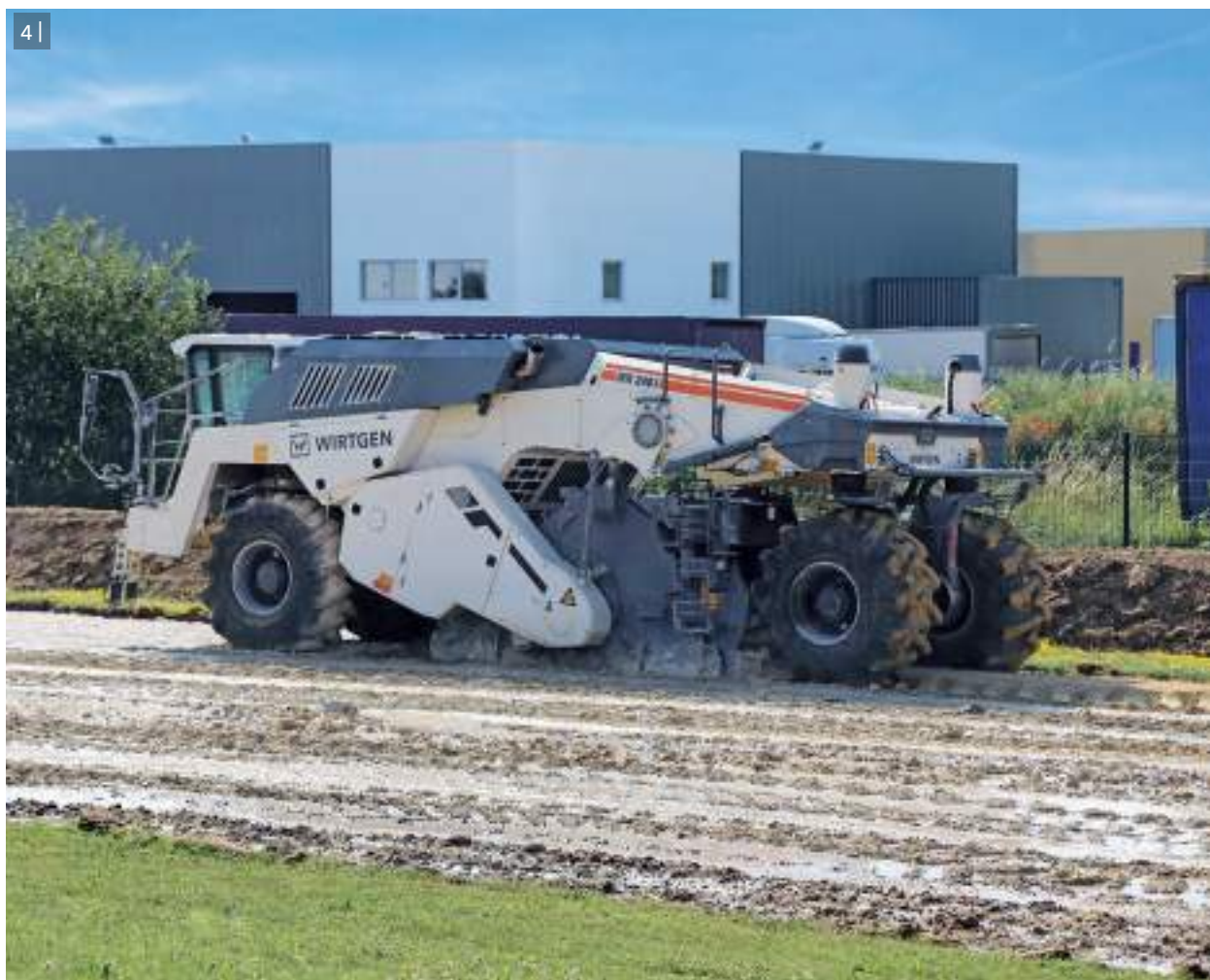
1 - 4 | Soil stabilization involves transforming sub-bases with insufficient bearing capacity into soil that is perfect for paving and compaction.
